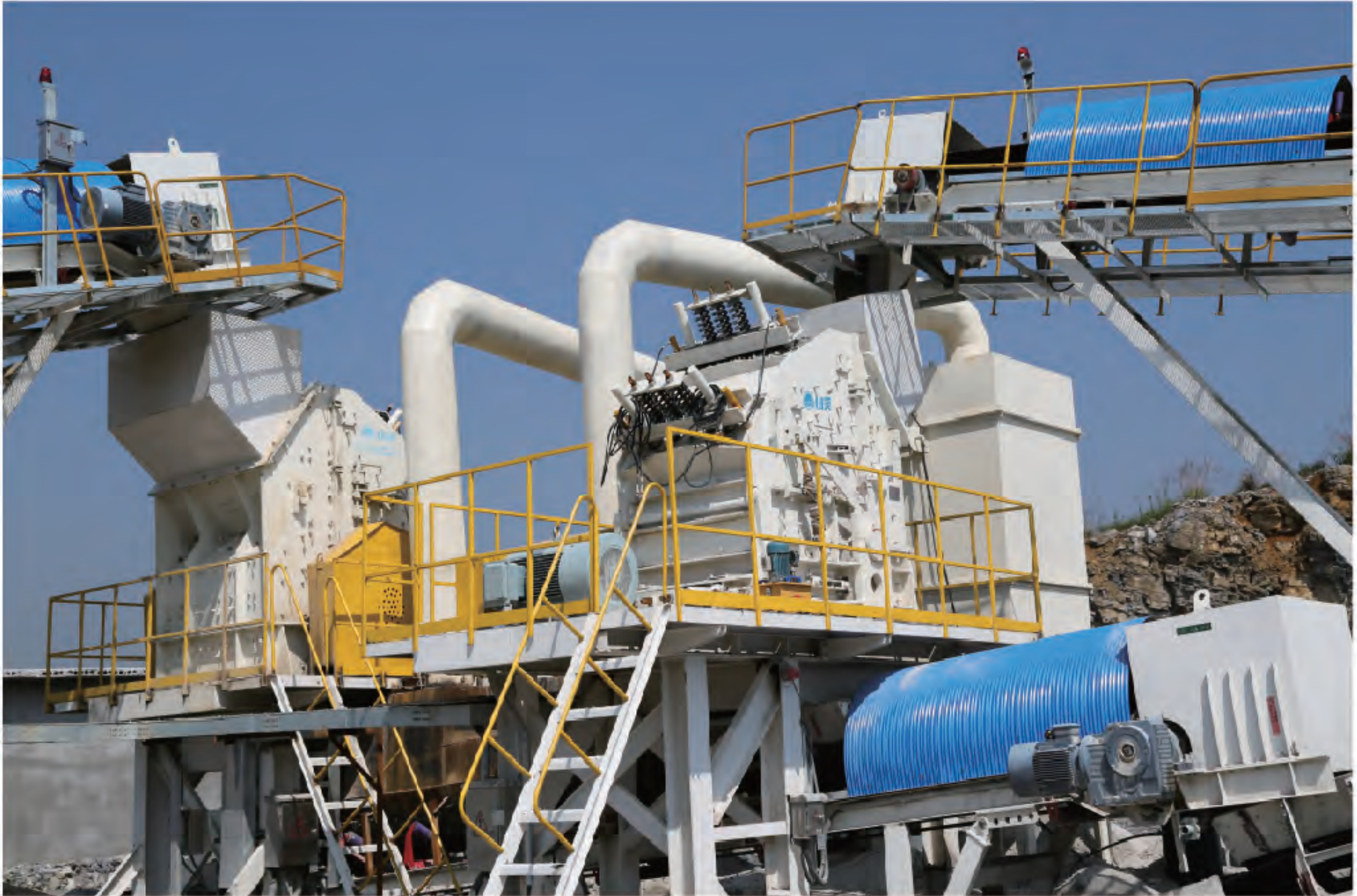
贵州拉法基项目现场 Lafarge Project in Guizhou
